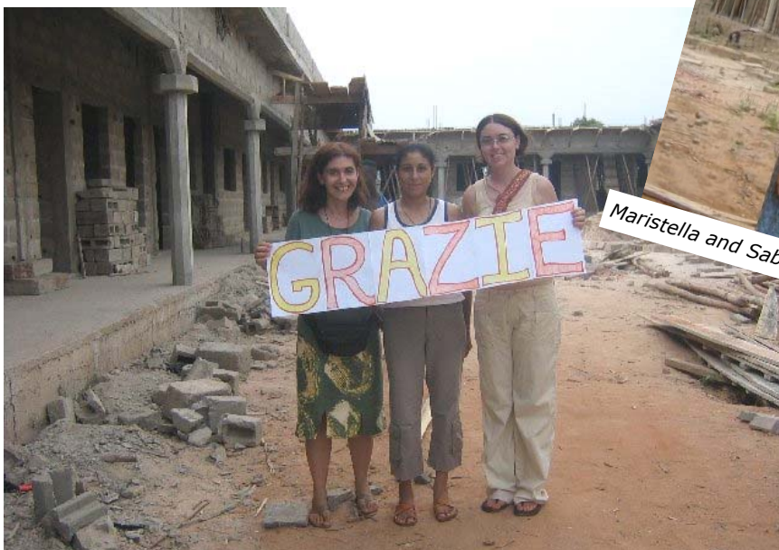
Maristella, Claudia, and Meghan express their gratitude to donors for the Togo dispensary (under construction in the background).
